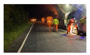
On the A2, four sections, each comprising of a 45mm surface course and varying from 700 to 1,000 lane metres in length, were carried out as part of the National Highways – A2 Kingston Scheme. They are:
